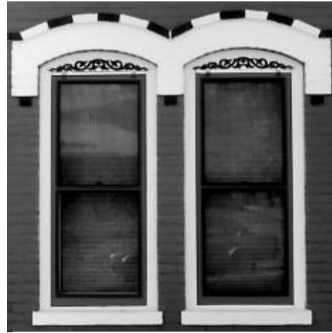
If a storm window is to be installed on the exterior, match the sash design of the original window (as this one does).
